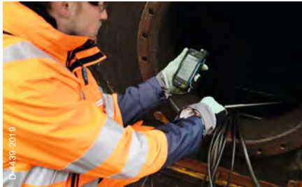
Entry into confined spaces/clearance measuring
